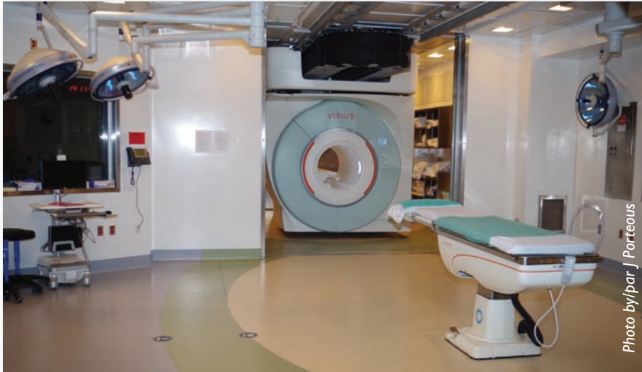
Theatre shielded doors are open to reveal the MRI magnet in its storage area.
