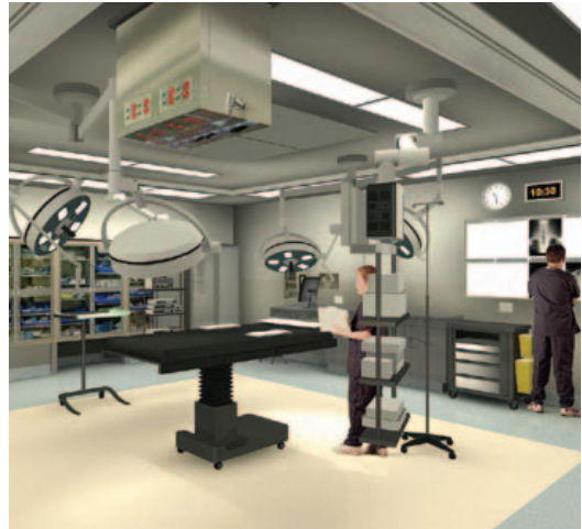
Double articulated boom systems in Digital OR Suite, University of Alberta Hospital.
